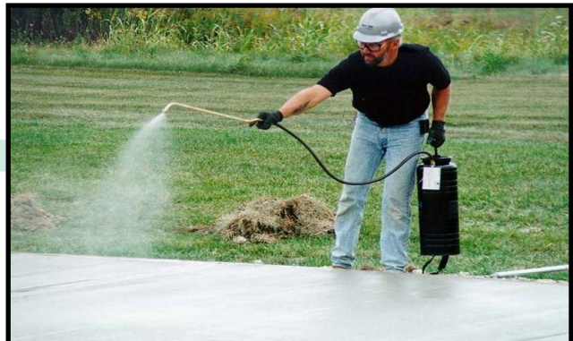
Spray-on curing compound
